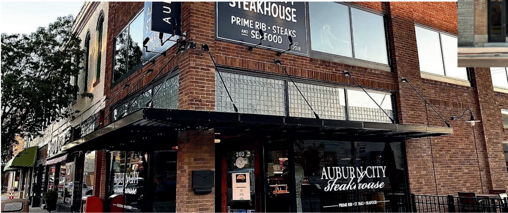
Auburn City Steakhouse occupies an 1859 building that operated as a hardware store for more than 150 years and changed ownership only four times.
